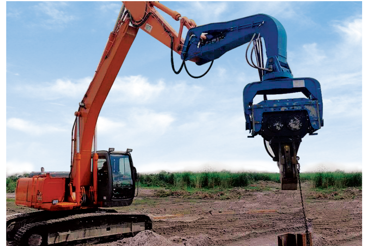
挖机锤施工案例 Excavator Mounted Vibro Hammer Construction Cases
